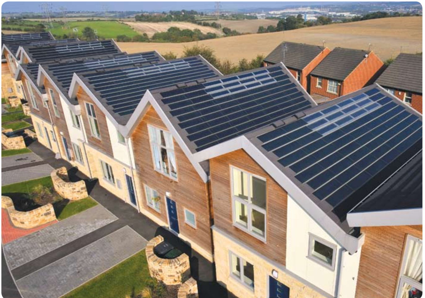
Solar roofs, Rothham, South Yorkshire
