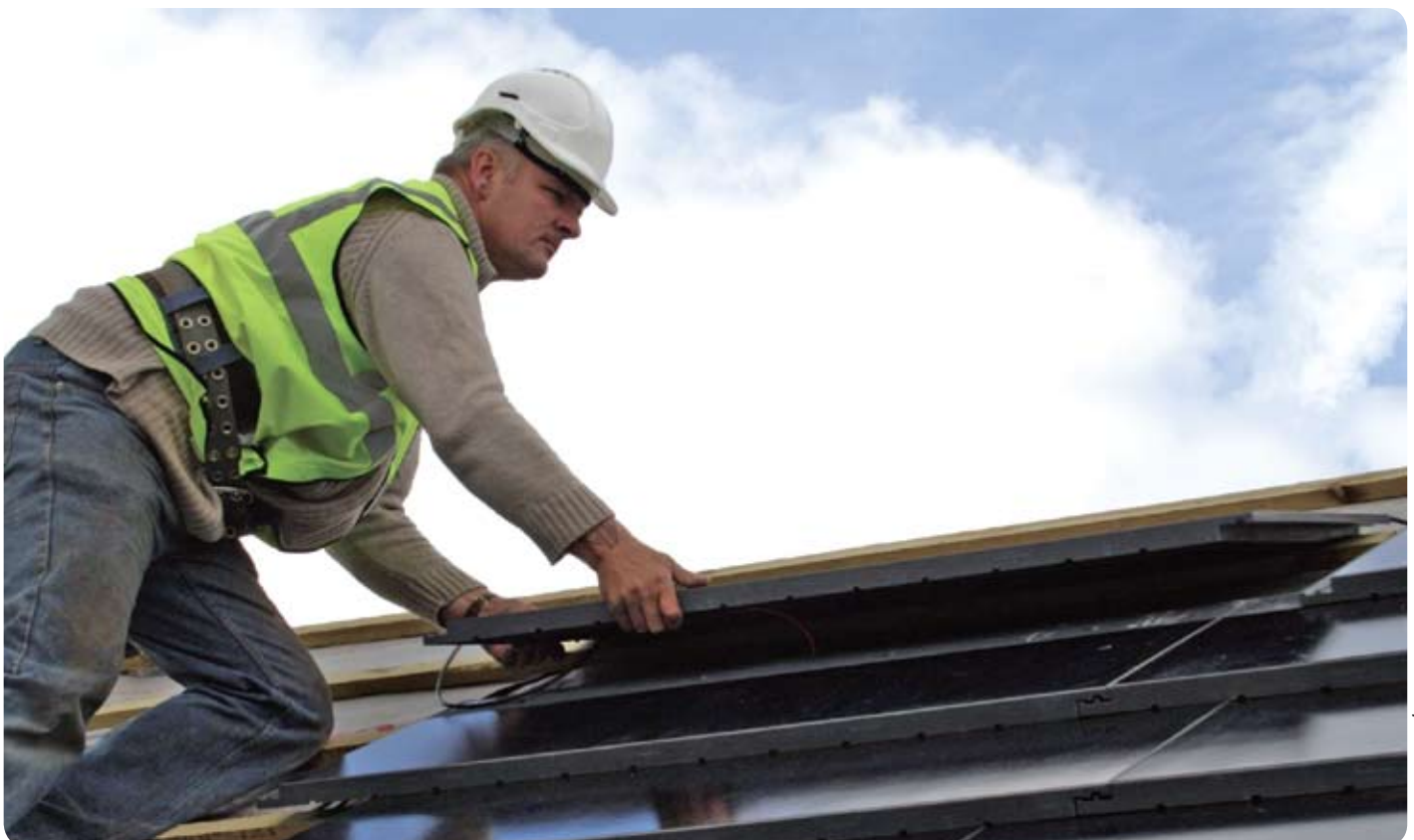
Solar roof tile installation, Melton Mowbray, Leicestershire
