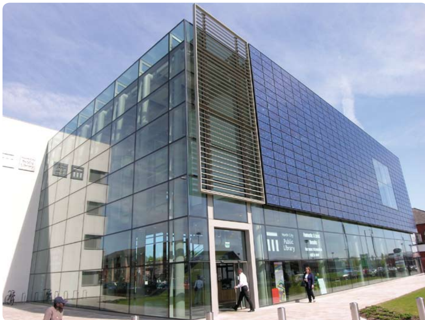
Solar facade, Manchester College of Art & Technology
